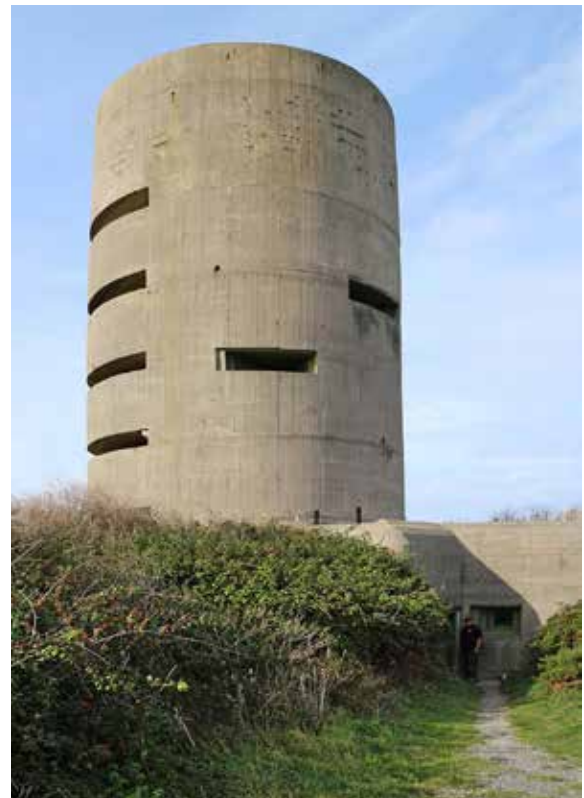
MP3 was built in 1942. The top three levels were used by the navy for their batteries. The two lower levels were taken over by the army for their two batteries of 22cm guns
